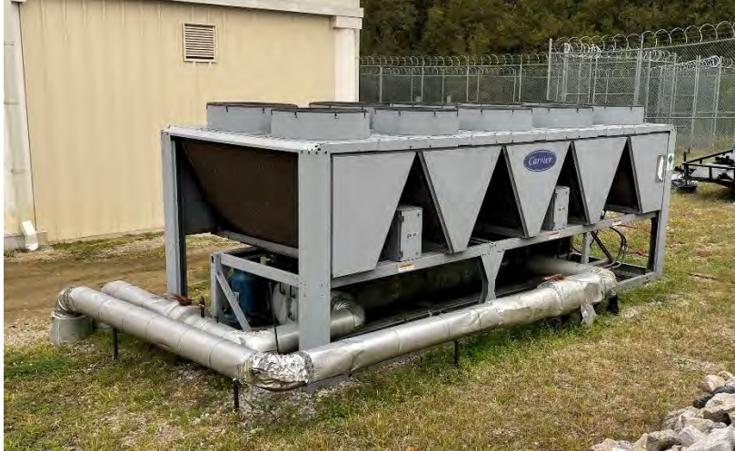
Photo 1: Air-Cooled Chiller
