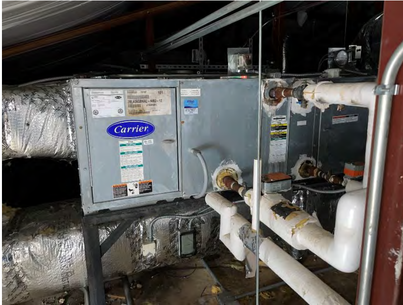
Photo 5: 4-Pipe AHU
